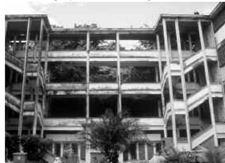
Fig. 4. Lycée Schœlcher, catwalks and flights of stairs
